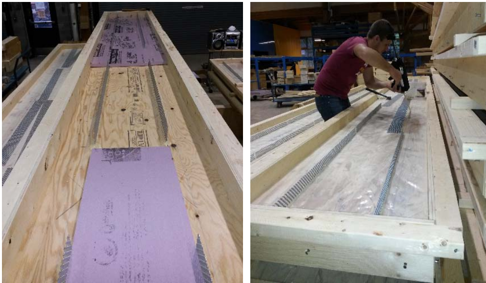
Figure 13: Installation of HBV mesh
